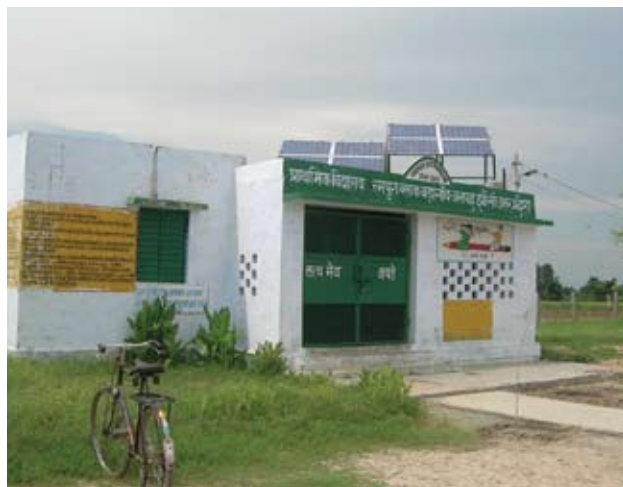
Rooftop solar panels in rural India.
